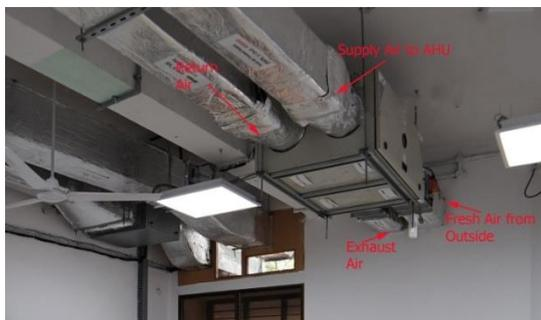
Figure 2 Photograph of Experimental setup
